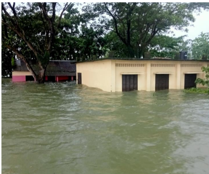
Photo: A flood-affected school in Sylhet that remains completely unusable until the water recedes. Photo taken by: Md. Abdul Awal, Companiganj, Sylhet.
